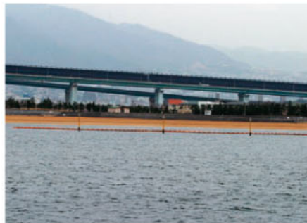
Thin piers standing in front of a beach.
