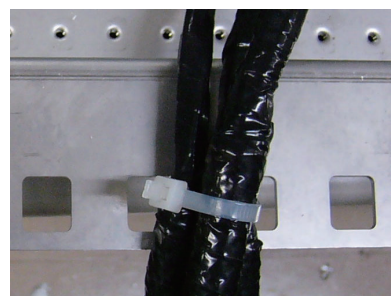
Fix cables to post with cable tie
